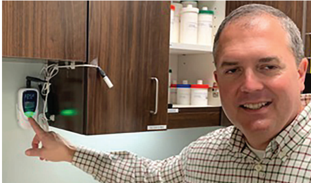
W-200 electronic temperature and humidity sensors monitor the pharmacy refrigerators and freezers
